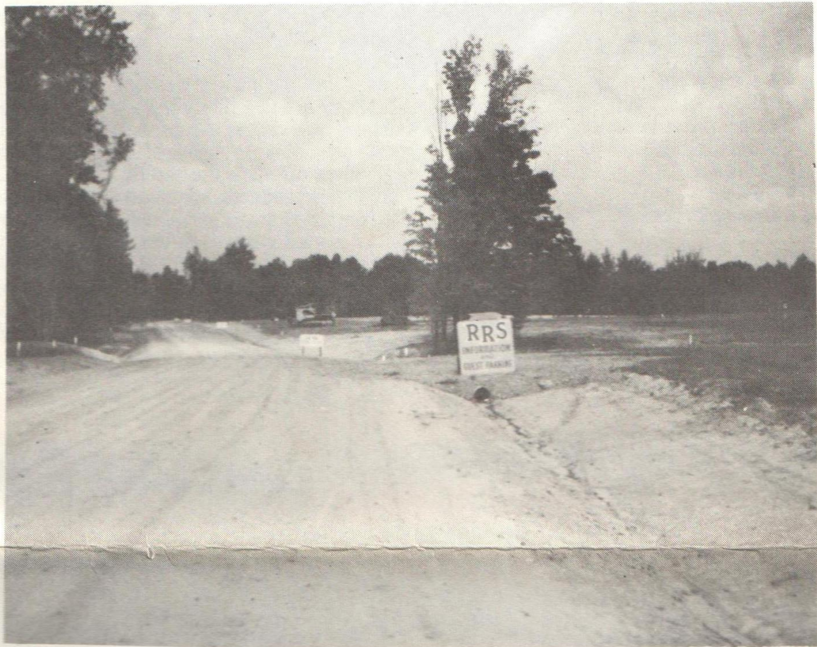
New construction at south end of Morning Star Drive.
