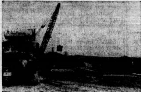
Heavy equipment pours concrete into forms on the west spillway.
