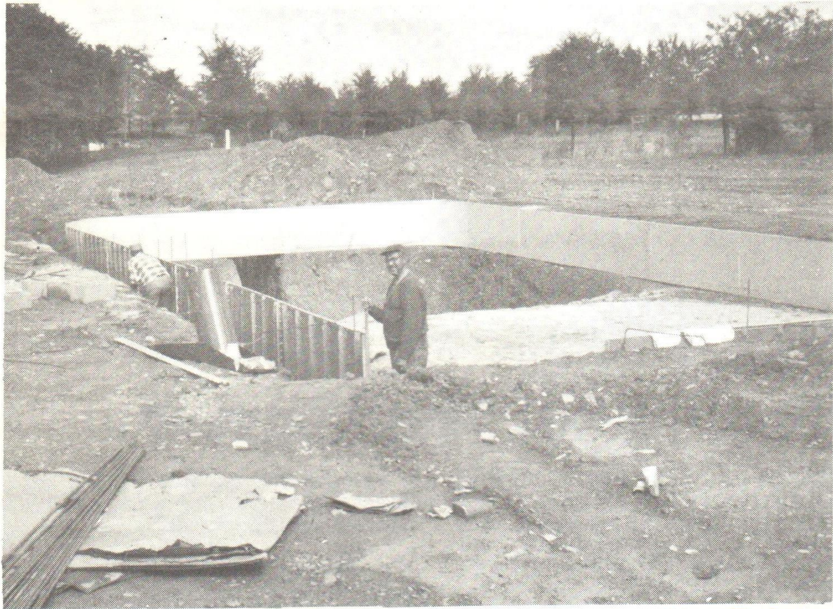
Construction starts on No. 4 pool--Morning Star Drive.
