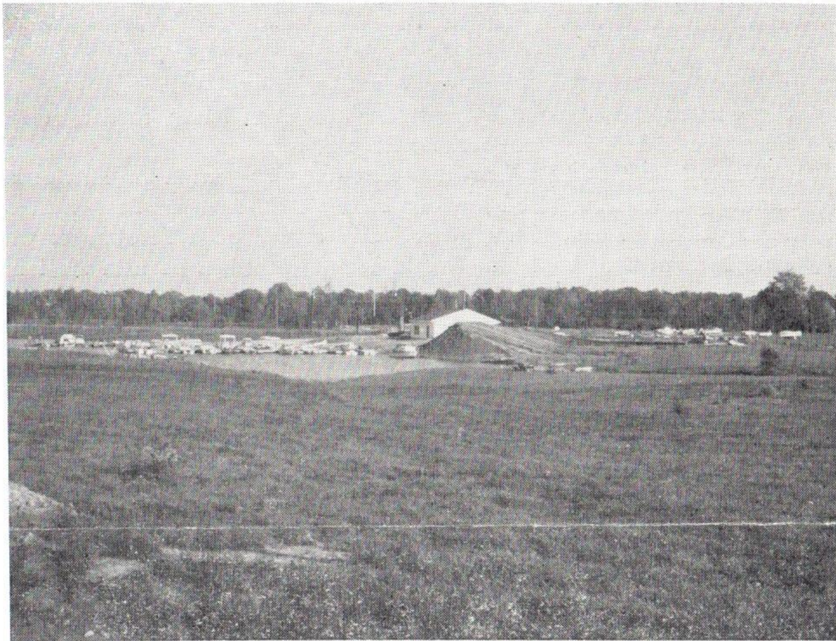
Construction of boat storage building started at Marina
