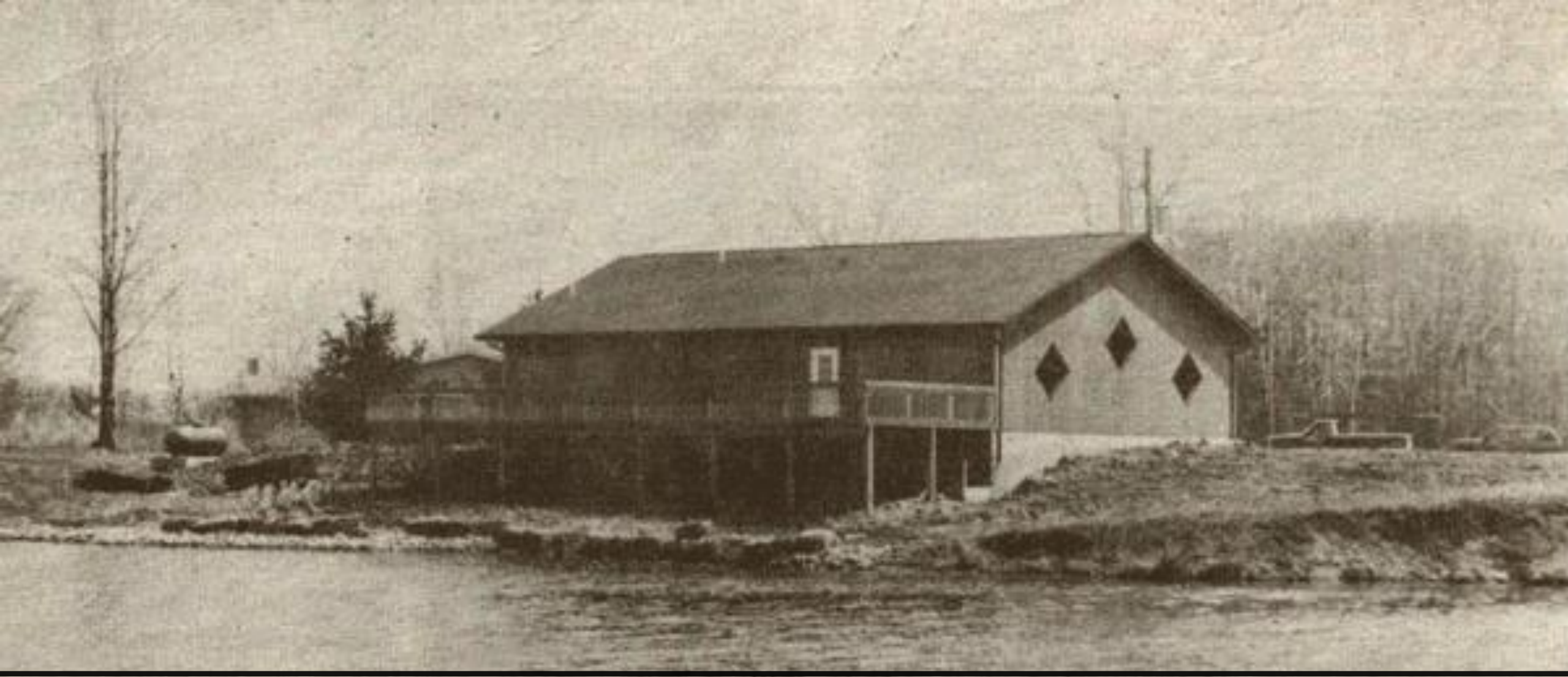
Construction of Marina Bay Café Now Paradise Bay
