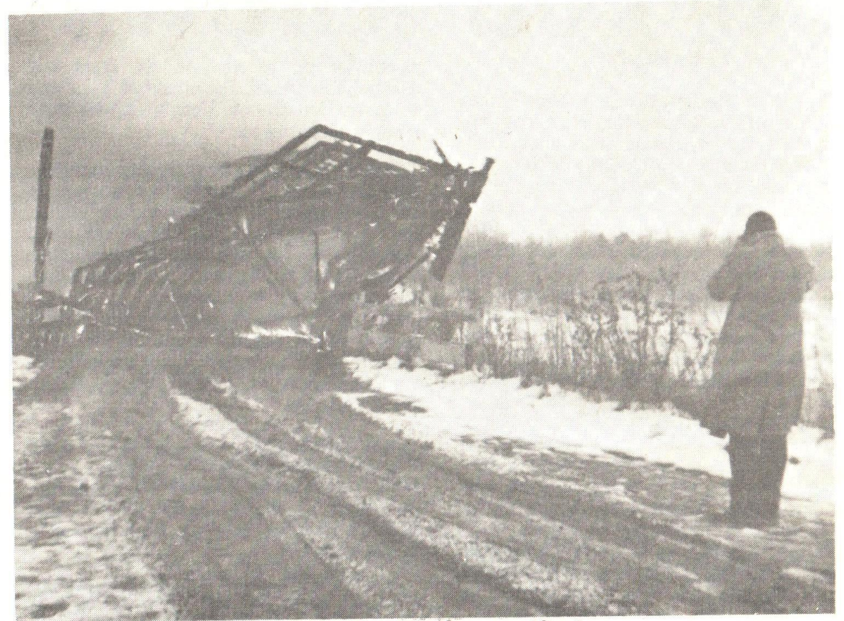
Calender Road Bridge - - - After!
