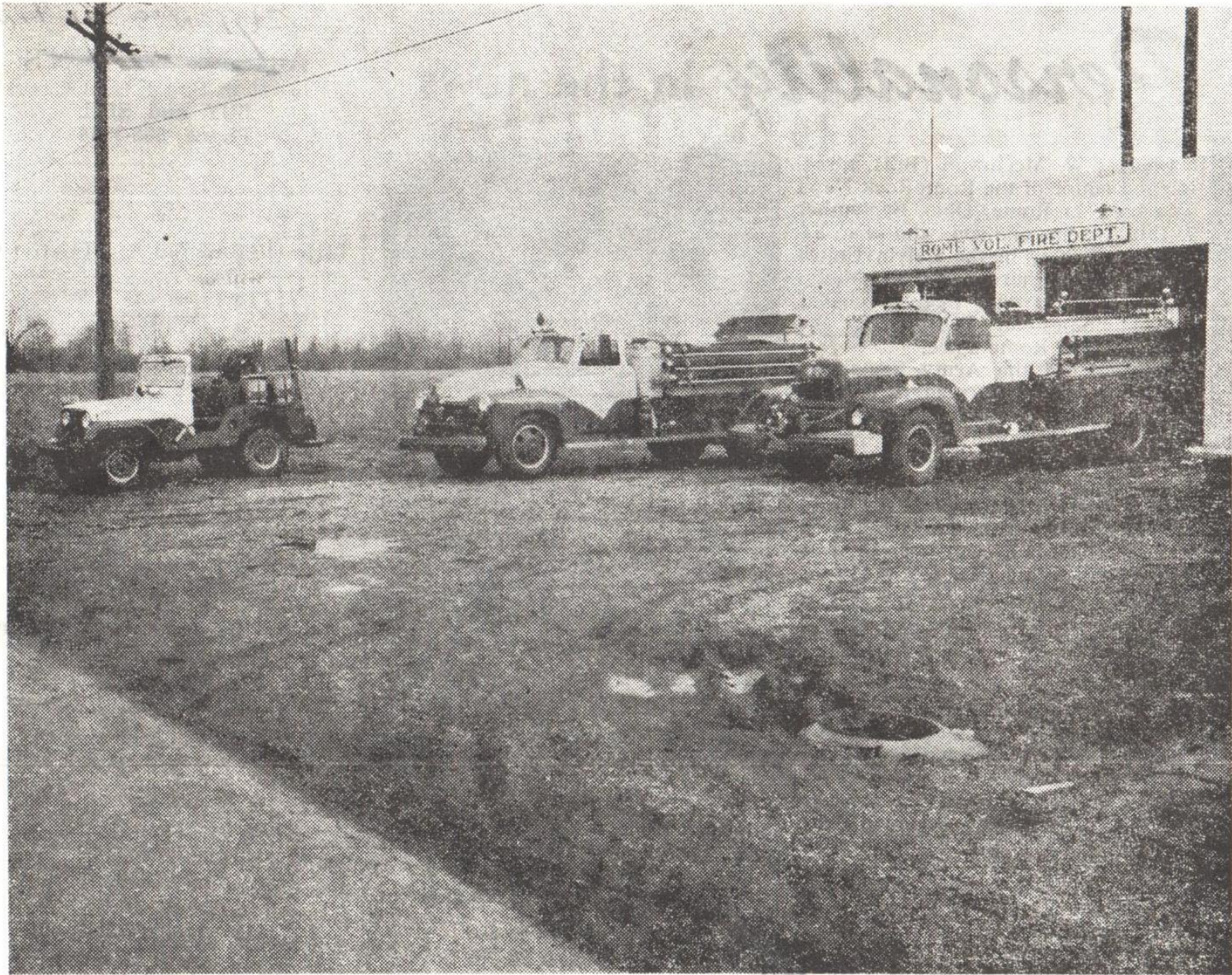
Units of the Rome Volunteer Fire Department
